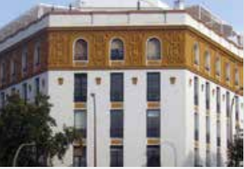
SOLIMPEKS Solar SL. SEVILLE / SPAIN
